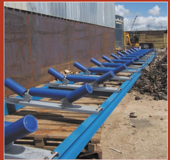
Polymer rollers being installed at Sims Metals.
